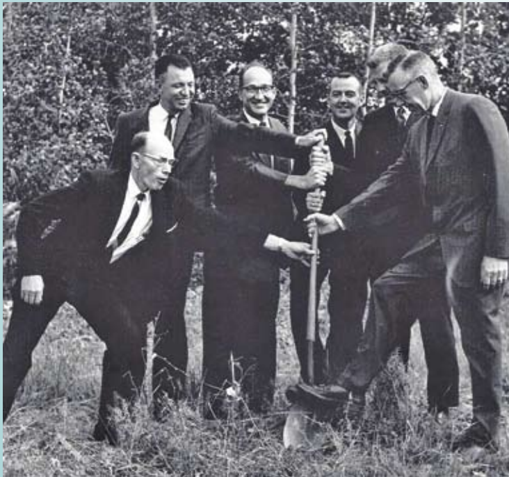
Highfields groundbreaking. Alton Stroud, superintendent of schools; Warren Ritter, juvenile court writer; Bob Drake, Highfields founder; Derwood Boyd, county supervisors (commissioners) representative; Al Beuerle, service club representative; and Joe Hicks, Area Building Trades Council.
